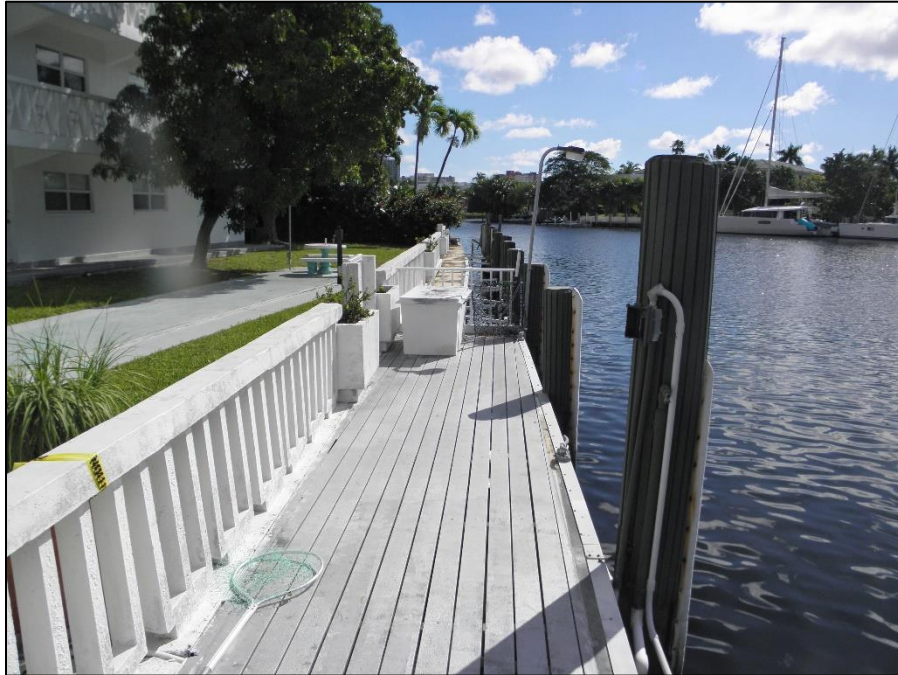
Photograph 4 Seawall on west side of property.
